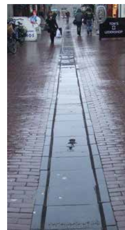
1. Goot over boulevard
